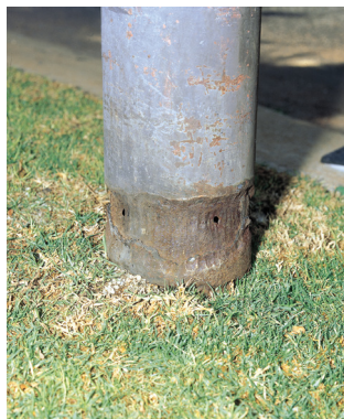
Corrosion of steel pole
